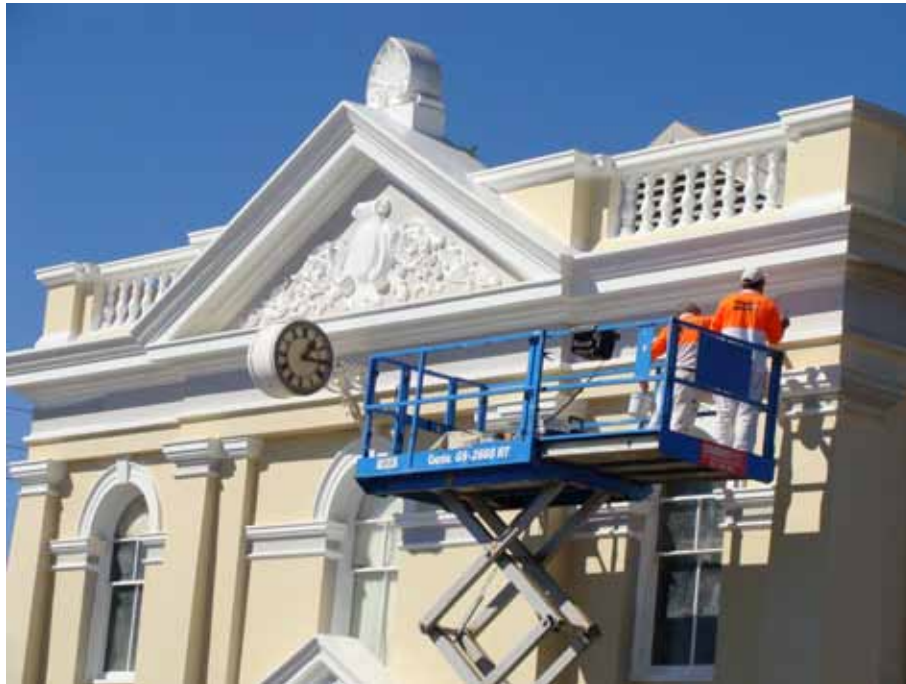
Refurbishment of the Geraldton Regional Art Gallery showing new colour scheme.
